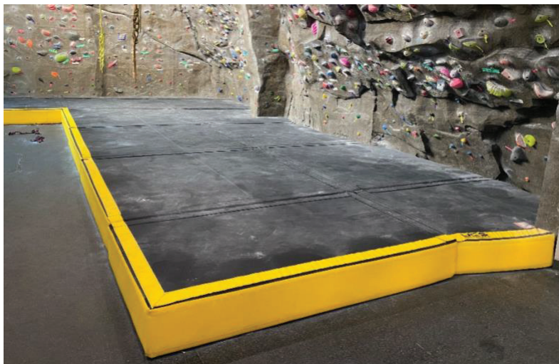
Finished Modular Boulder Padding System Installed.
